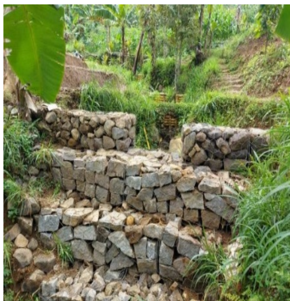
Gabion structure - during construction
